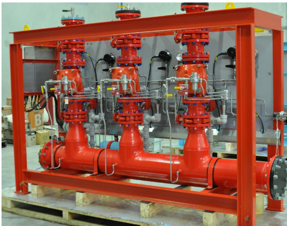
3 valve skid under test
